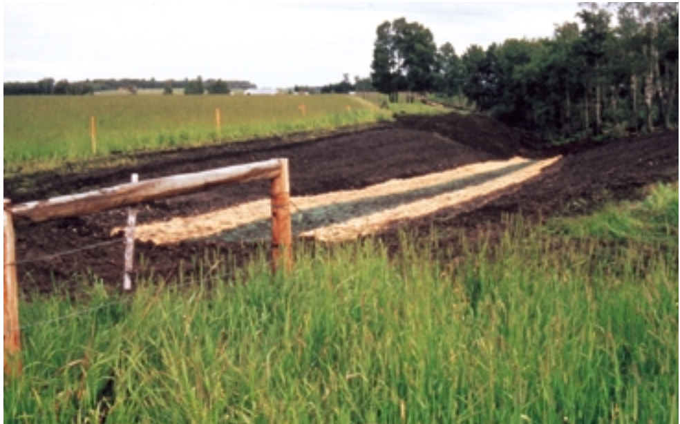
Figure 2.66 These erosion control methods slow the flow of water and enable trees and shrubs to take root in the gully again.
