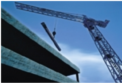
Figure 4.67A A heavy mass acts as a counterweight to keep the crane stable.
