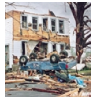
Figure 4.42 Winds in a tornado produce twisting, bending, and compression forces so strong that no structure can escape damage.
