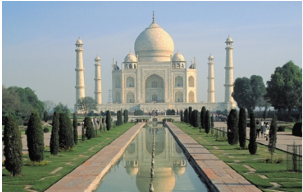
Figure 4.7 The dome of the Taj Mahal in Agra, India, is one of the most famous shell structures in the world.
