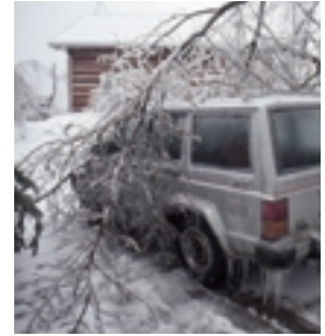
Figure 4.16 Extreme weather conditions can cause both natural and manufactured structures to fail.
