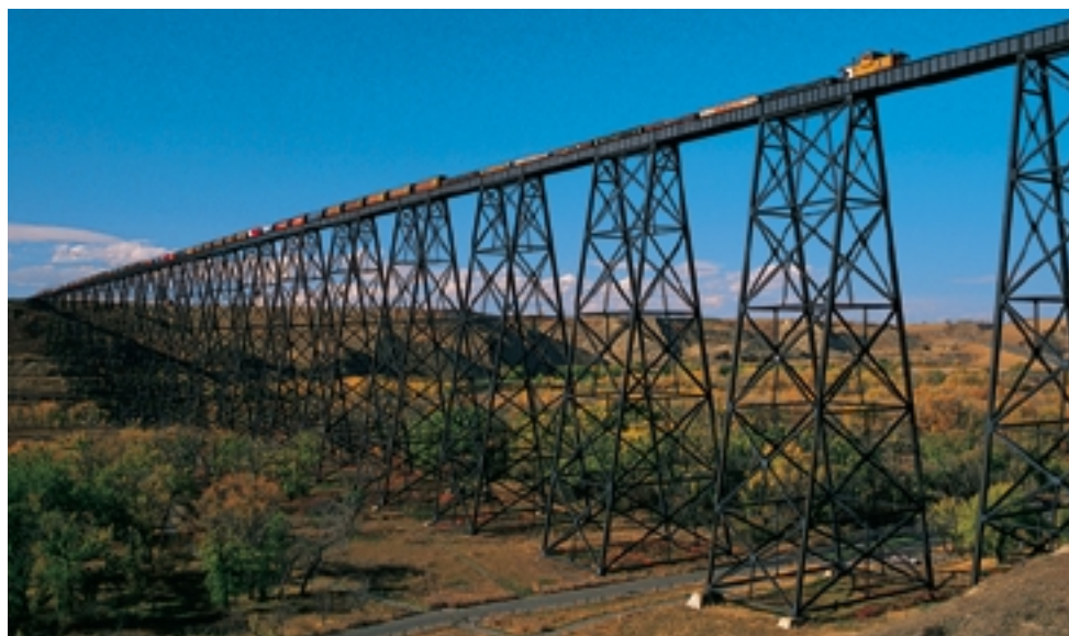
Figure 4.12 This trestle bridge in Lethbridge, Alberta, was the longest structure of its height in the world when it was built in 1909. It carries trains 97 m above the valley of the Oldman River, for a distance of 1.6 km.
