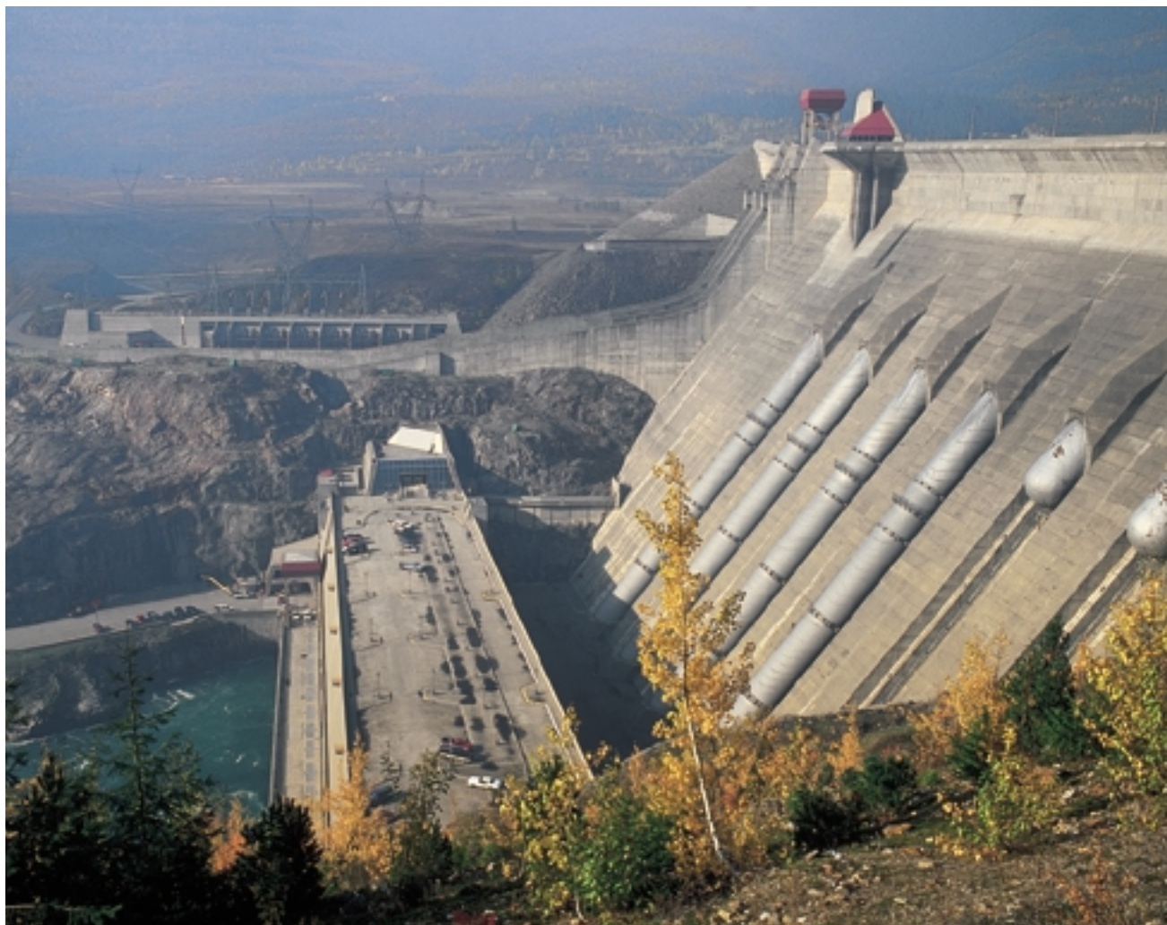
Figure 3.29 Dams use the energy of falling water which is transformed into electrical energy.
