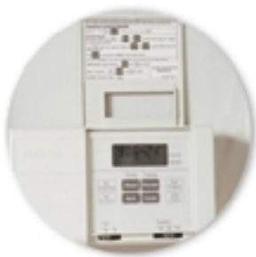
Figure 3.40 Programmable thermostats can be set to adjust the temperature so that a home is cooler when its occupants are away or sleeping.
