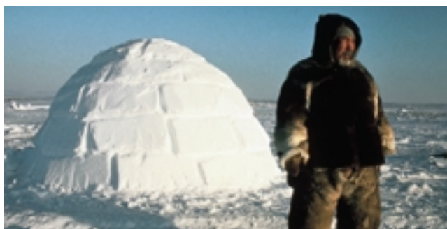
Figure 3.1E This Inuit hunter has built an igloo shelter. When he perspires inside the igloo, the moisture will condense when it hits the ice, sealing the igloo.
