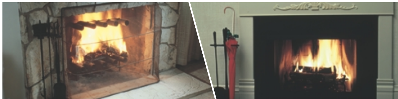
Figure 3.1B Open wood-burning fireplaces (at right) draw the warmth from a room. Modern gas fireplaces (above) use energy efficiently, directing warm air back into the room.
